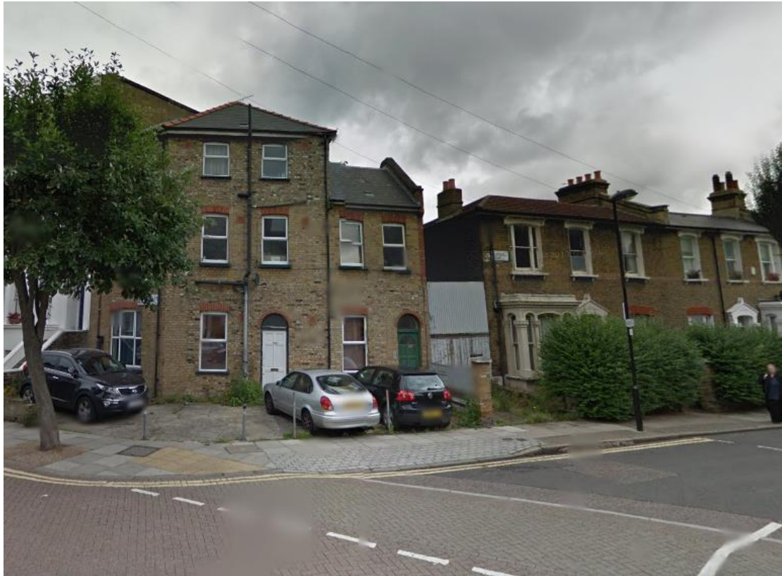
Photo 3: Subject site on right prior to commencement of existing works
